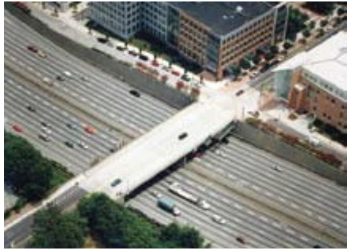
5th Street Bridge Before Improvements (Source: Aspire Magazine)
